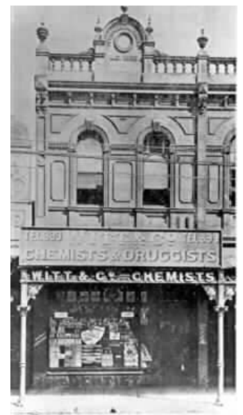
Pickford's pharmacy in High Street, Armadale. The business continued to trade under the name of William Witt, who had established a pharmacy 25 years before in another location
