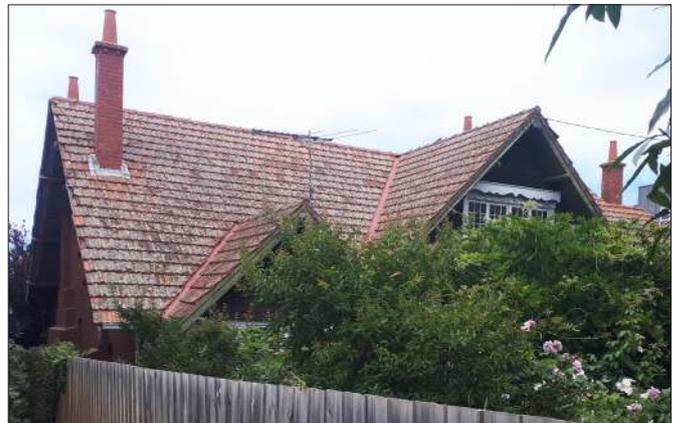
Number 380 showing the roof clad in terracotta Marseille pattern tiles and tall red brick chimneys with corbelled capping and terracotta pots. The central dormer four-bay window is clad with stained timber shingles. An off-centre receded entry porch with double timber doors is at ground level.<sup>6</sup>
